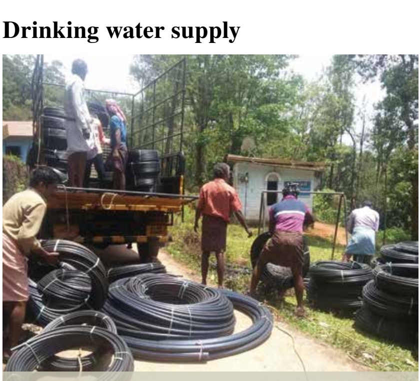
Distribution of pipes for channeling drinking water from natural springs: Rs.132000/-
